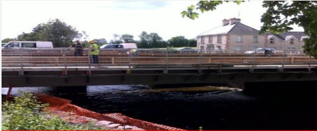
Bridge deck, Northern Ireland
